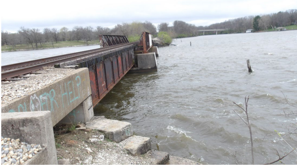
Figure 1 - Side view of Gilman Sub CN Bridge near Toronto, IL
