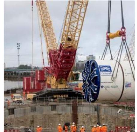
Tunnel Boring Machine (TBM)
