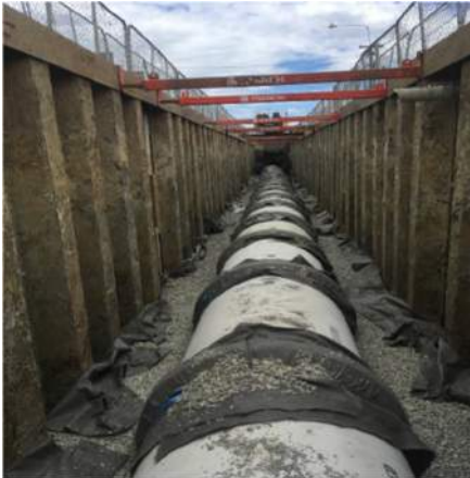
Trenching "Cut and Cover"
