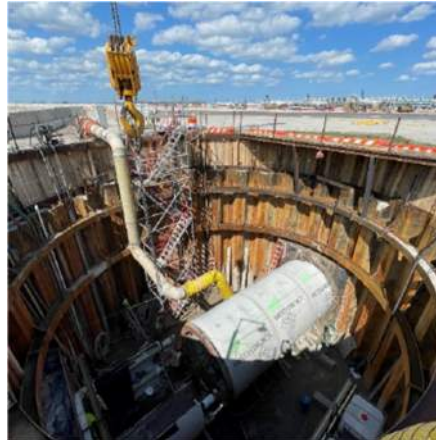
Microtunnel Boring Machine (MTBM)
