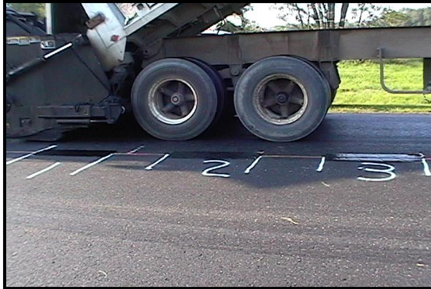
Figure 24: IL 40 Paving over Joint Sealant Formulations
