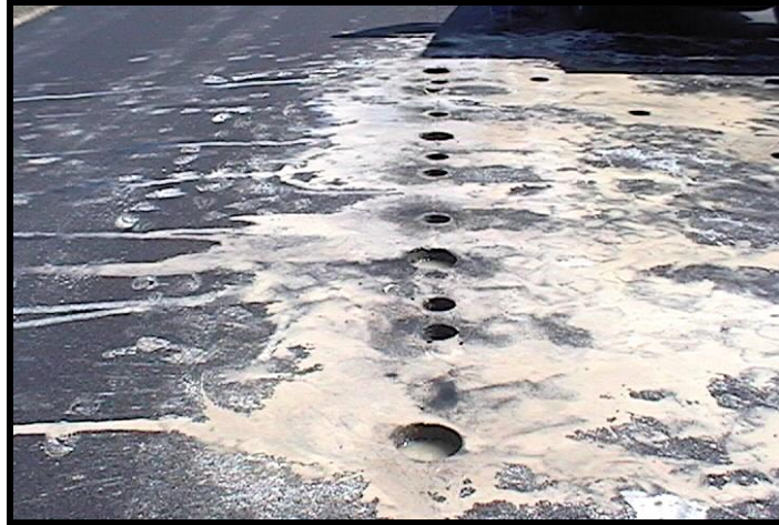
Figure 25: IL 40 after Coring Test Locations
