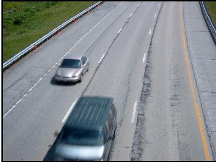
Figure 2: Cold Joint
