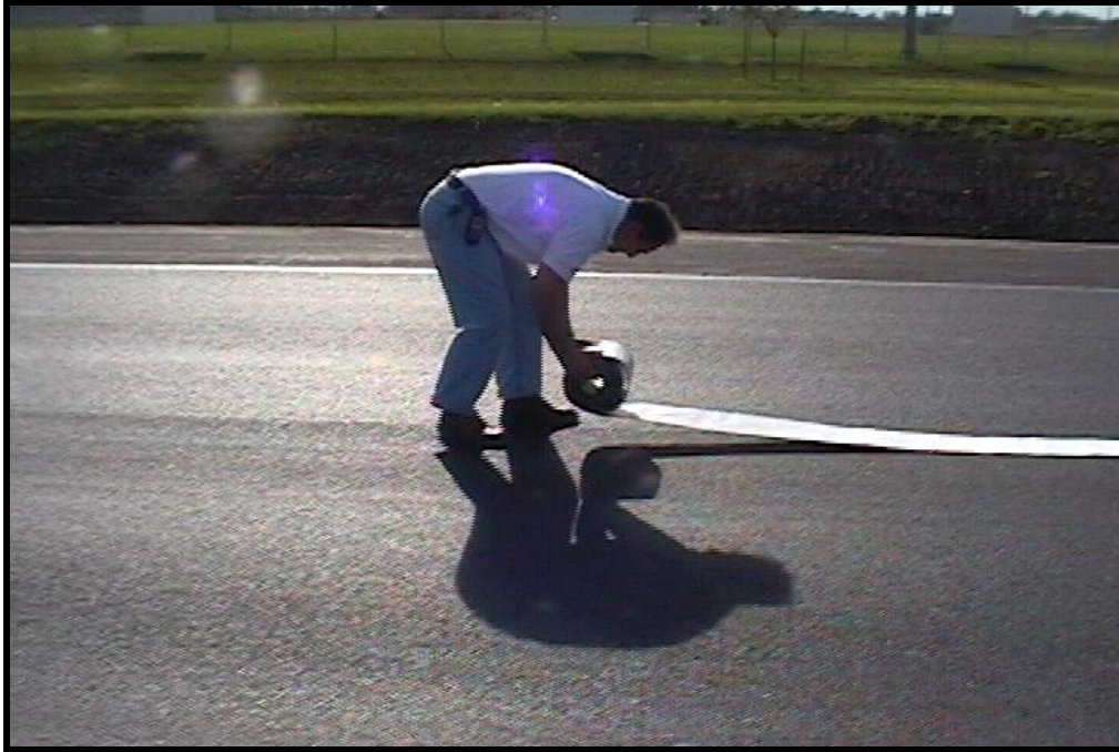
Figure 41: US 51 QuikSeam Placement
