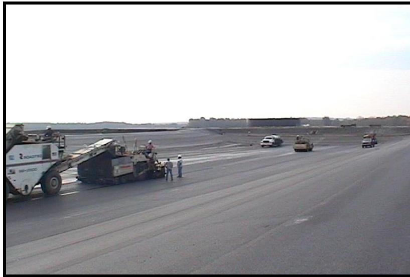
Figure 29: Retention Pond Paving
