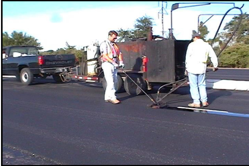
Figure 39: US 51 Jband Placement
