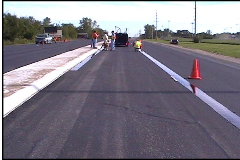
Figure 45: US 51 Jband Median Placement
