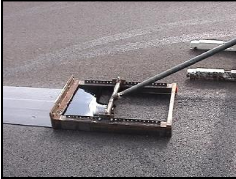
Figure 30: Jband Placement
