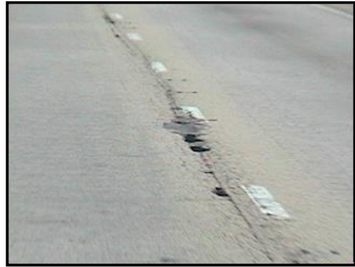
Figure 5: Low Joint Density Area
