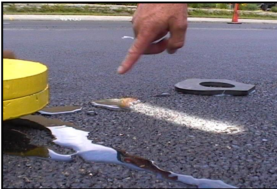
Figure 21: Field Permeameter Water Resurfaces along the Joint
