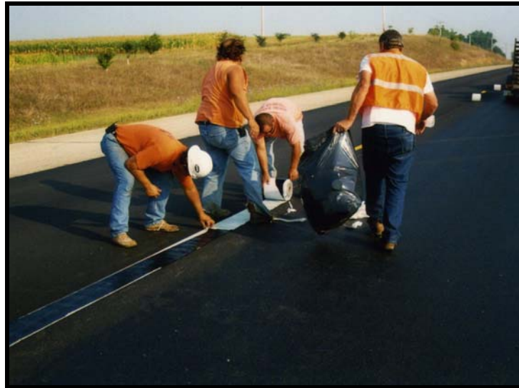
Figure 11 Removal of QuickSeam ® plastic backing
