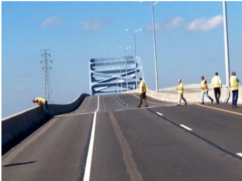
Figure 38. The obvious pavement sag sustained by the collapse of Pier 22 in October 2013 after 30 years of service of the I-43 tied-arch truss bridge over the Fox River in Green Bay, WI, necessitated an $8 million emergency repair. Photo source: Wisconsin DOT.
