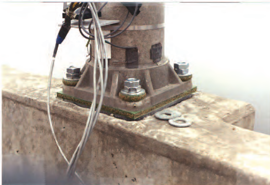
Figure 13. Preloading of the Airloc washers and pad, resulting in compression bulging of the polymer and cork interior.
