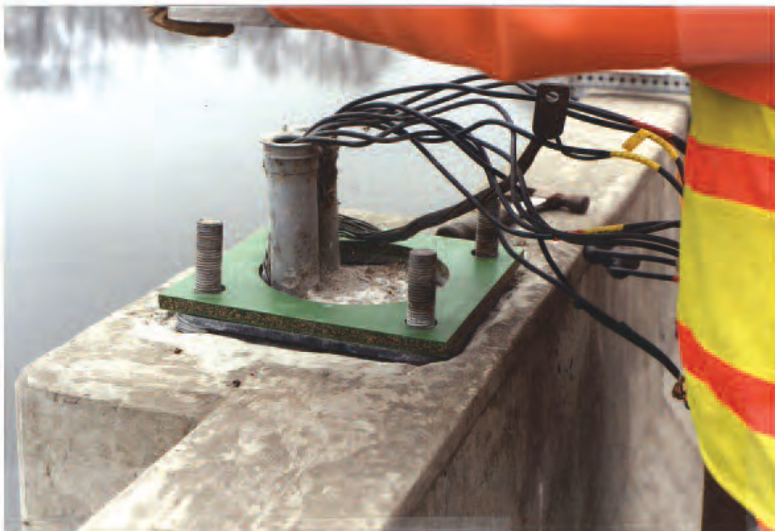
Figure 12. Installation of the Airloc pad by contractor personnel.
