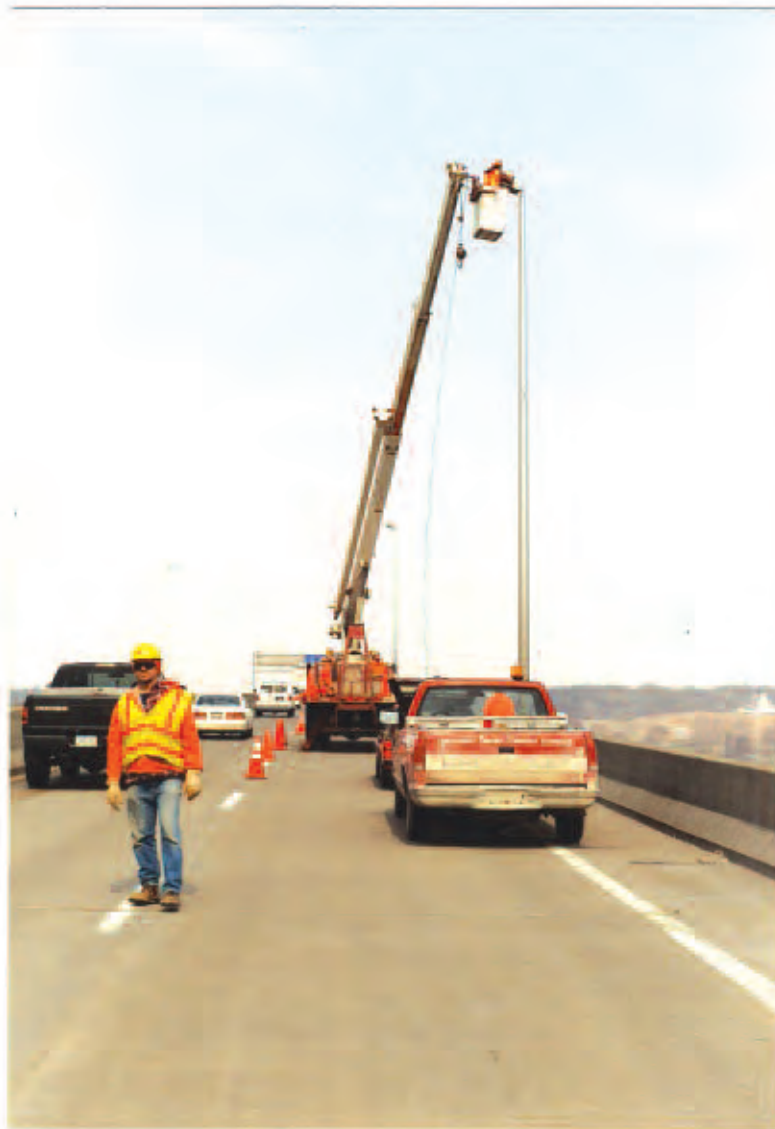
Figure 10. Installation of accelerometers on the luminaire on the poles mounted on the parapets of the Le Claire Bridge.
