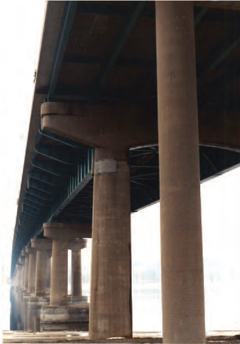
Figure 1. Photograph of the LeClaire Bridge over the Mississippi River, taken from the western approach, showing beam stringers of piers 8 and 9. The superstructures of the intermediate spans consist of two deep plate girders which support cantilevered floor beams. An 8-in thick reinforced slab deck, composite in the positive moment areas, rests on 24-in deep wide flange stringers.
