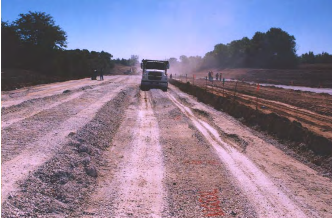
Figure 6. Loading Transition area between Type A (foreground) and Type B (background) CLS CA-6. Note edge effects the right side of the photo corresponding to the left wheel path
