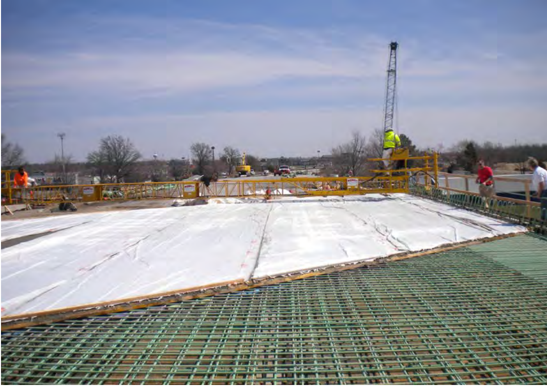
Photo 11: District 9 UltraCure placement
