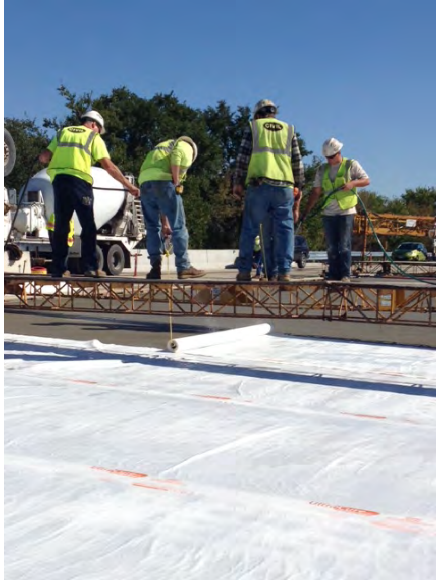
Photo 6: District 2. Rolling the UltraCure across the deck.
