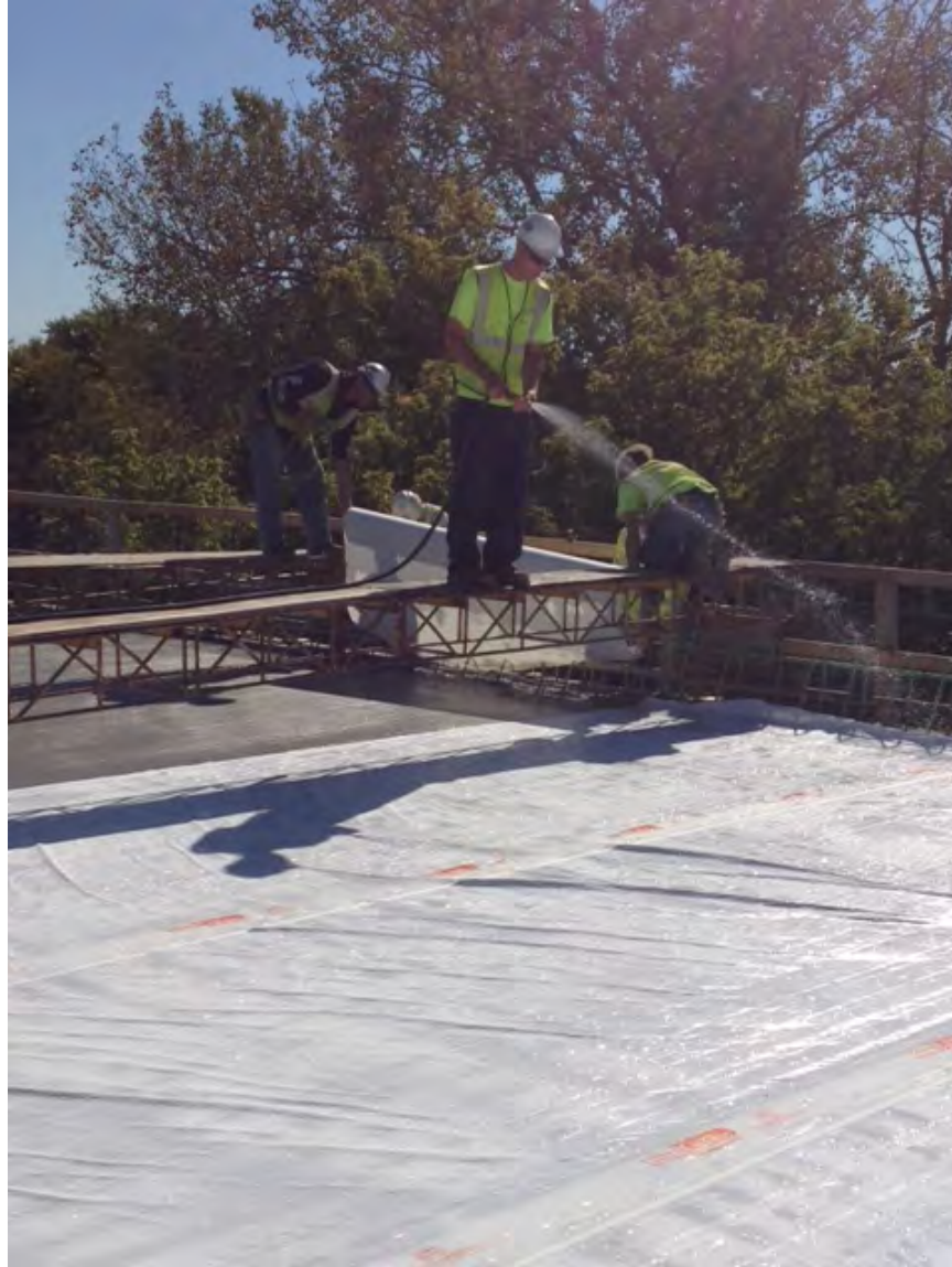
Photo 8: District 2. Spraying of water onto the surface of the UltraCure.
