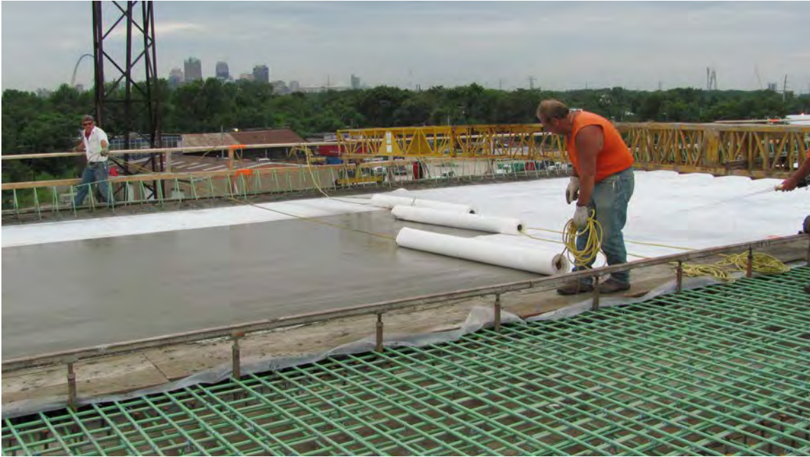
Photo 2: District 8. UltraCure mat being placed using the “wedding runner” method.
