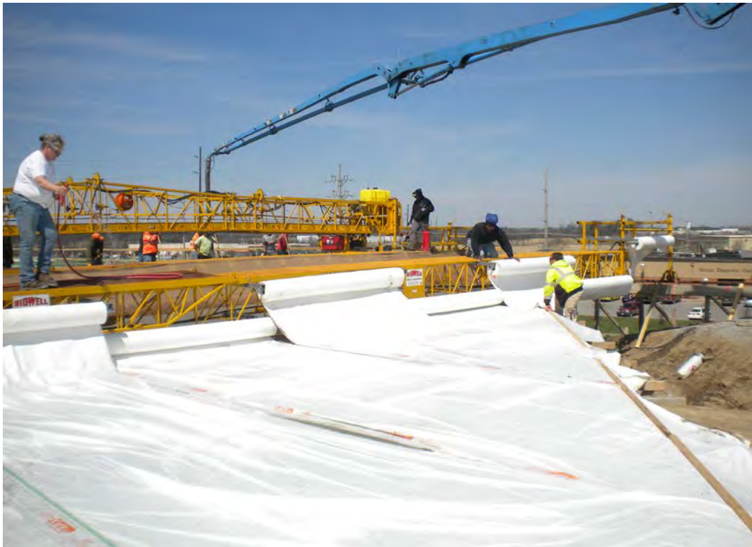
Photo 10: District 9 UltraCure placement
