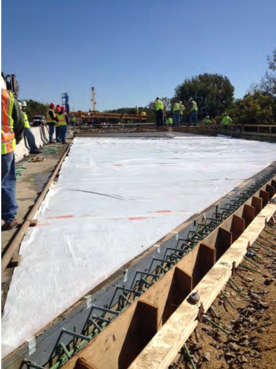
Photo 4: District 2. Hand placed UltraCure at the start of the skewed deck.
