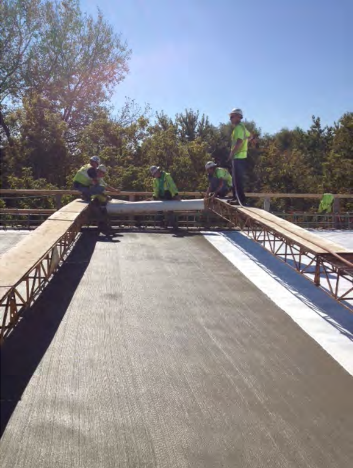
Photo 5: District 2. Preparing the UltraCure roll to be placed across the deck.
