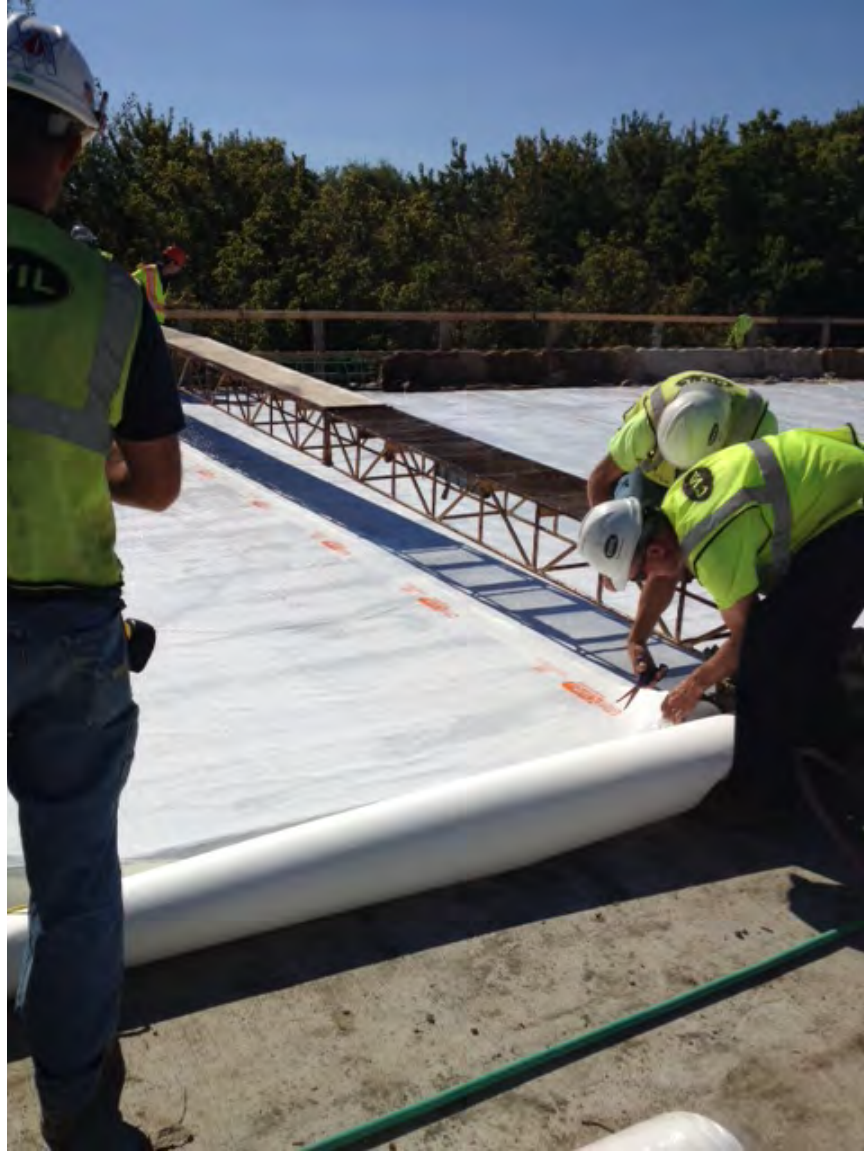
Photo 7: District 2. Cutting the UltraCure at the edge of the deck.
