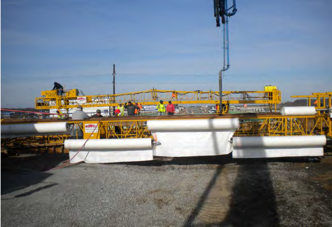
Photo 9: District 9 UltraCure placement
