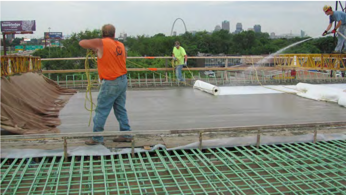
Photo 3: District 8. Spraying water on the UltraCure as it is rolled out.
