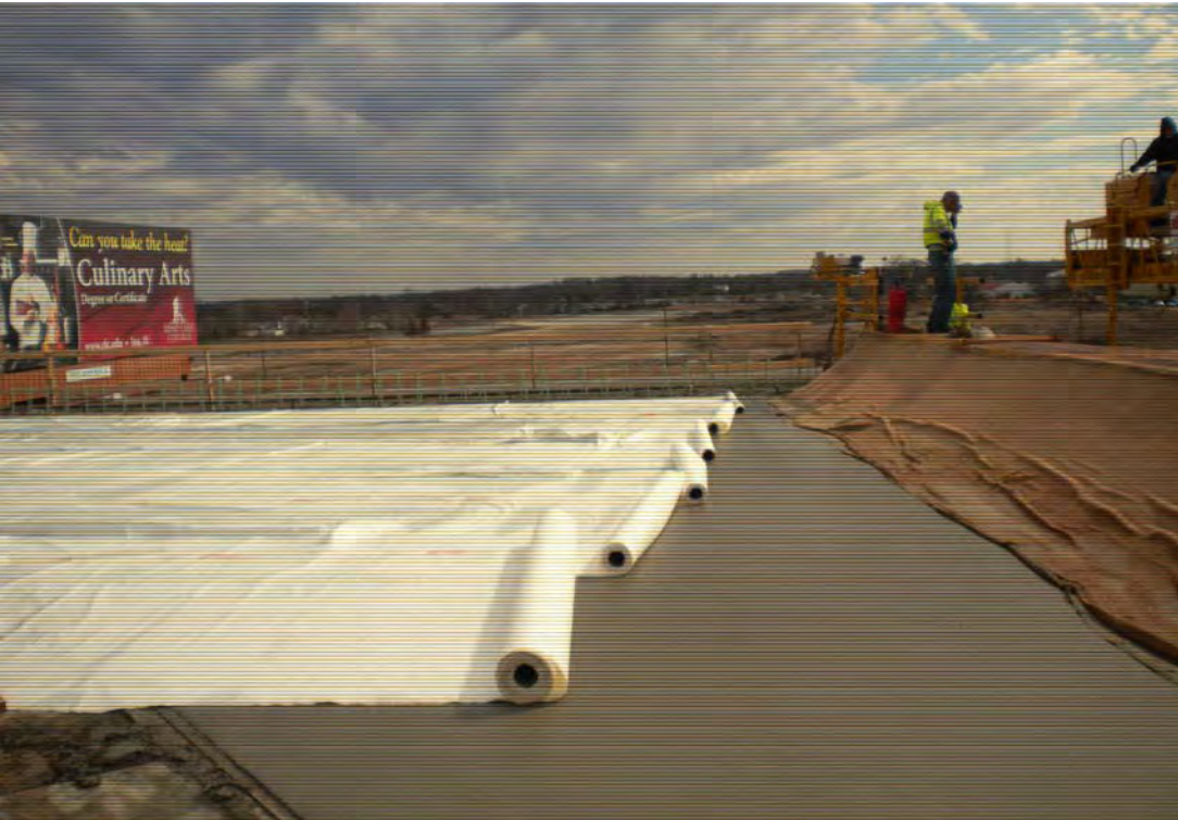
Photo 12: District 9 UltraCure placement
