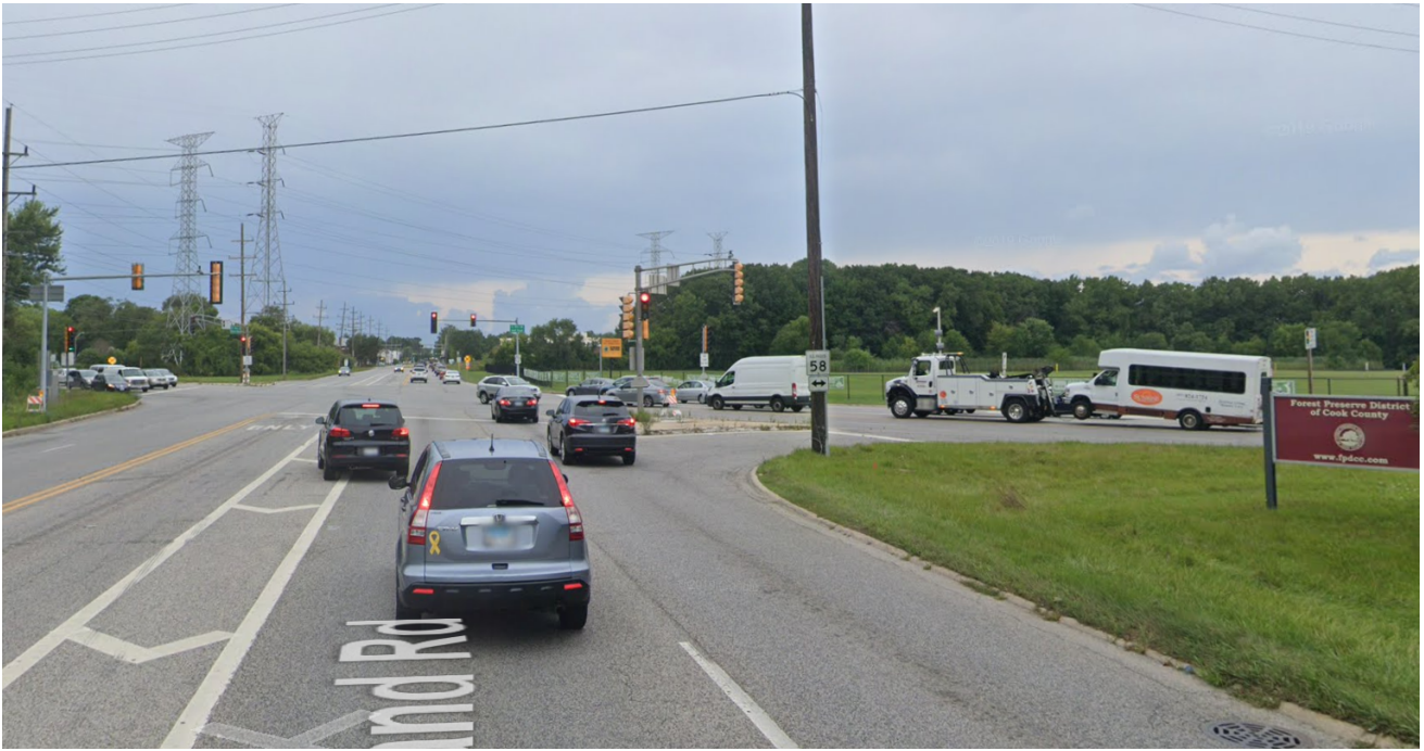
US 12 (Rand Road) south of IL 58 (Golf Road) facing northwest
