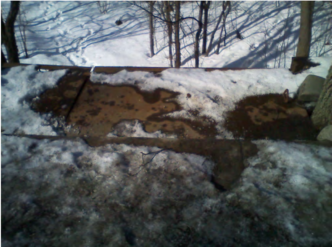
Location: Steel plate, west side.
