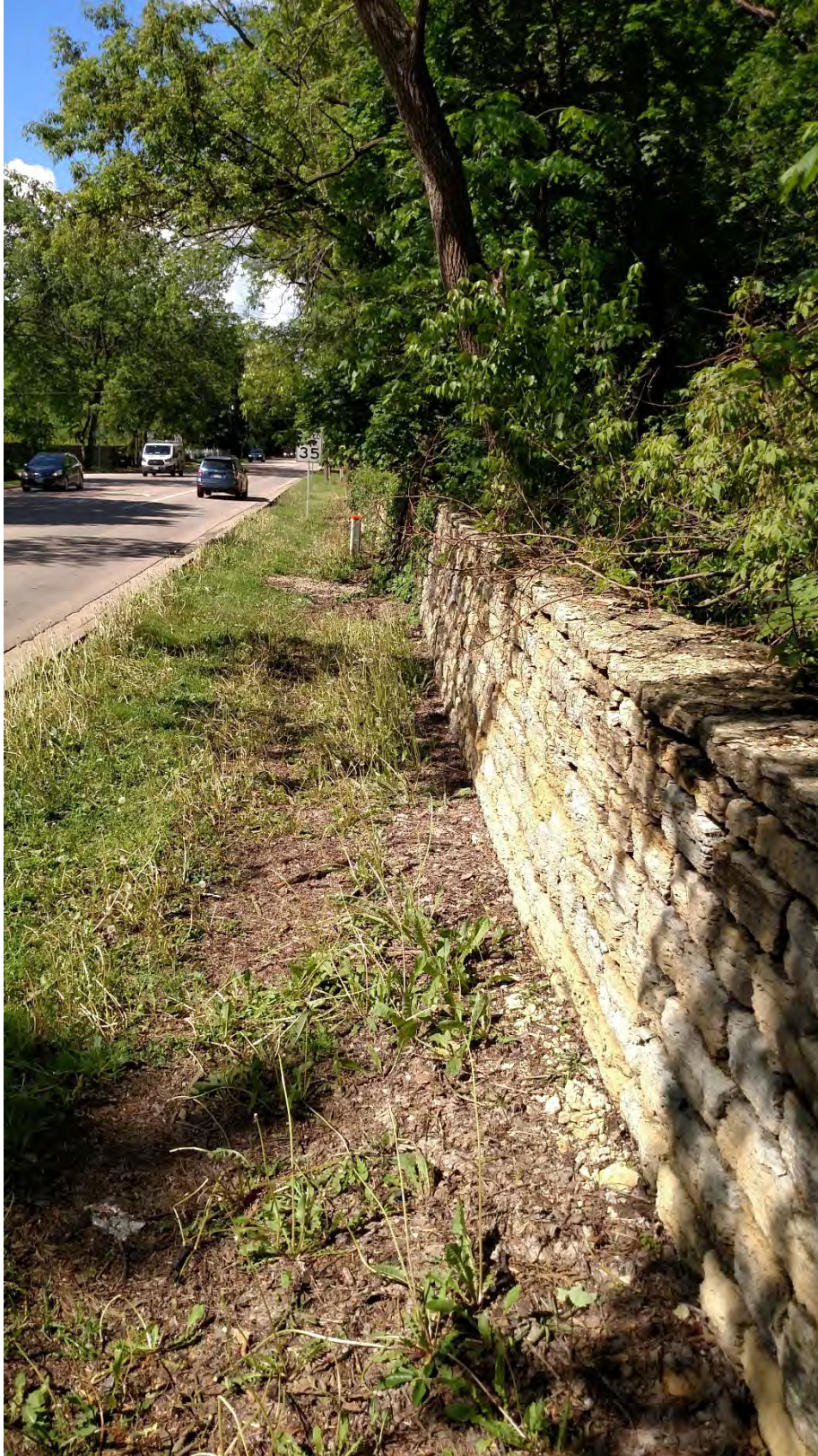
Location: Masonry Wall along IL 31 looking north
