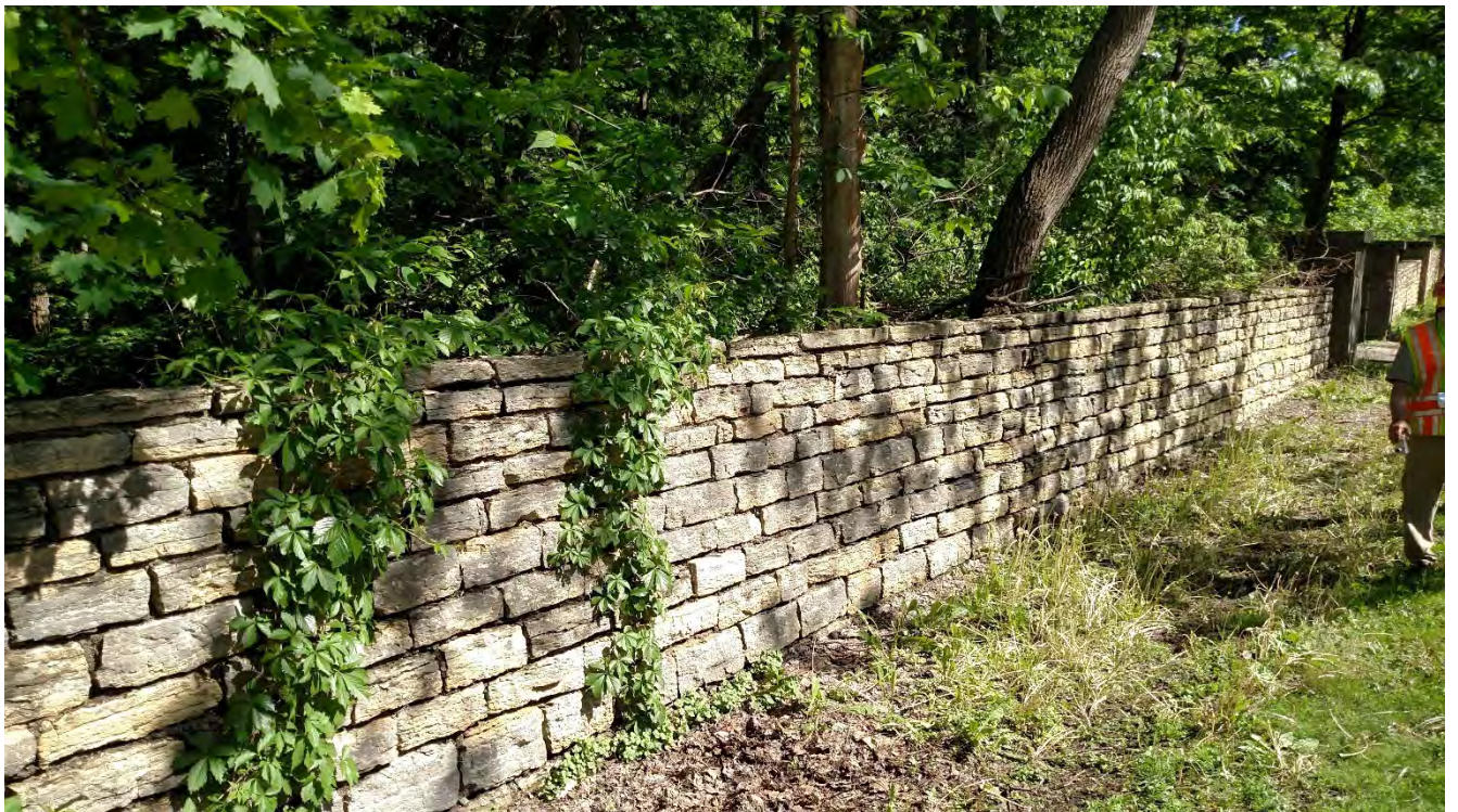
Location: Masonry Wall looking south
