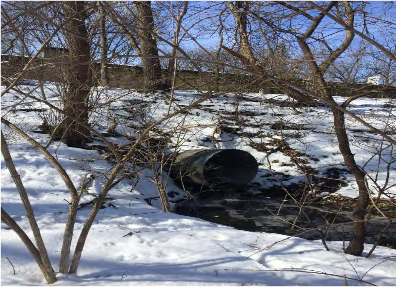
Location: East Structure.
