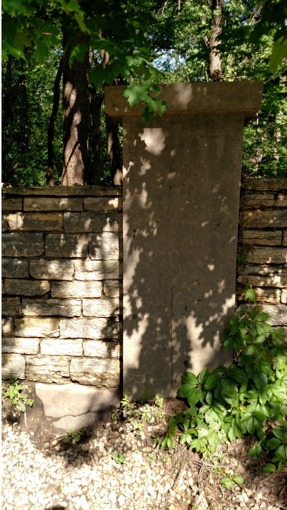
Location: Masonry Wall looking east
