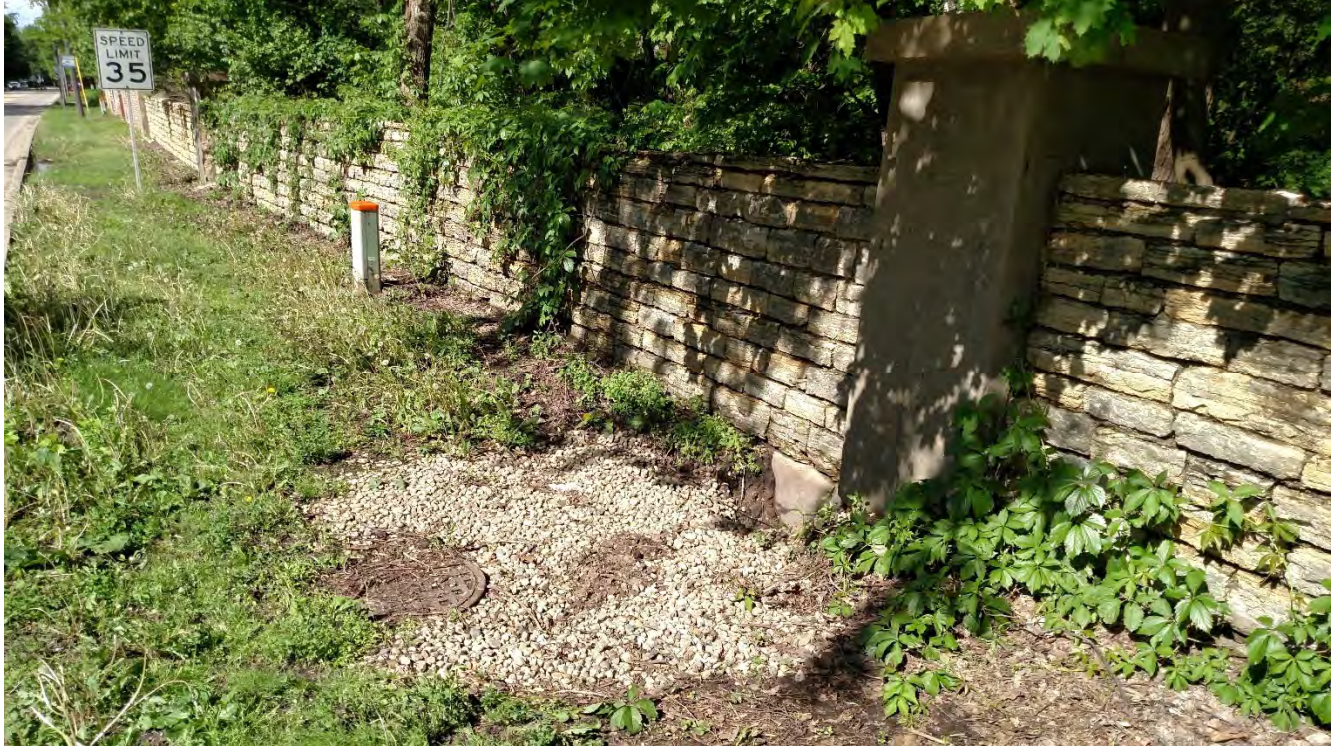
Location: Masonry Wall along IL 31 looking north
