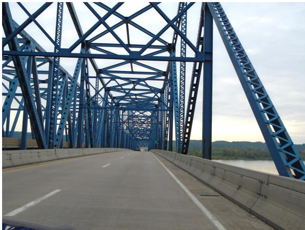
On main bridge span of eastbound US 150 facing east
