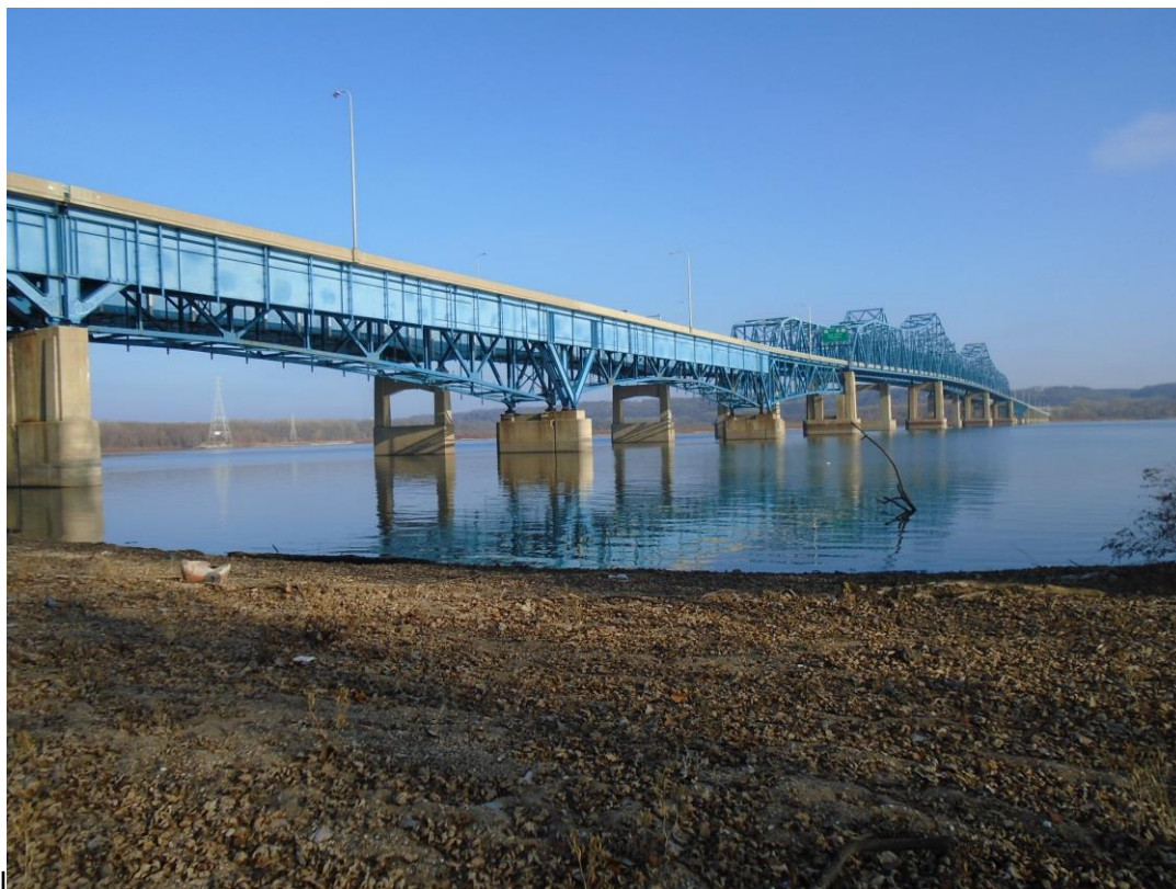
West side of the Illinois River facing east (eastbound structure on right)
