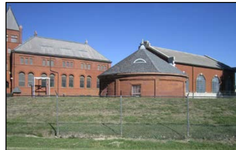
Peoria Waterworks (Photo by Jeff Bushur, 2014 site visit)
