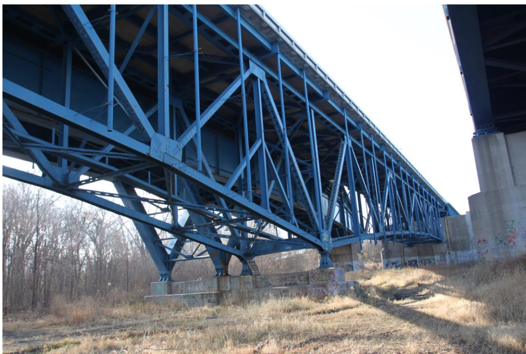
West abutment (eastbound bridge on left) facing west
