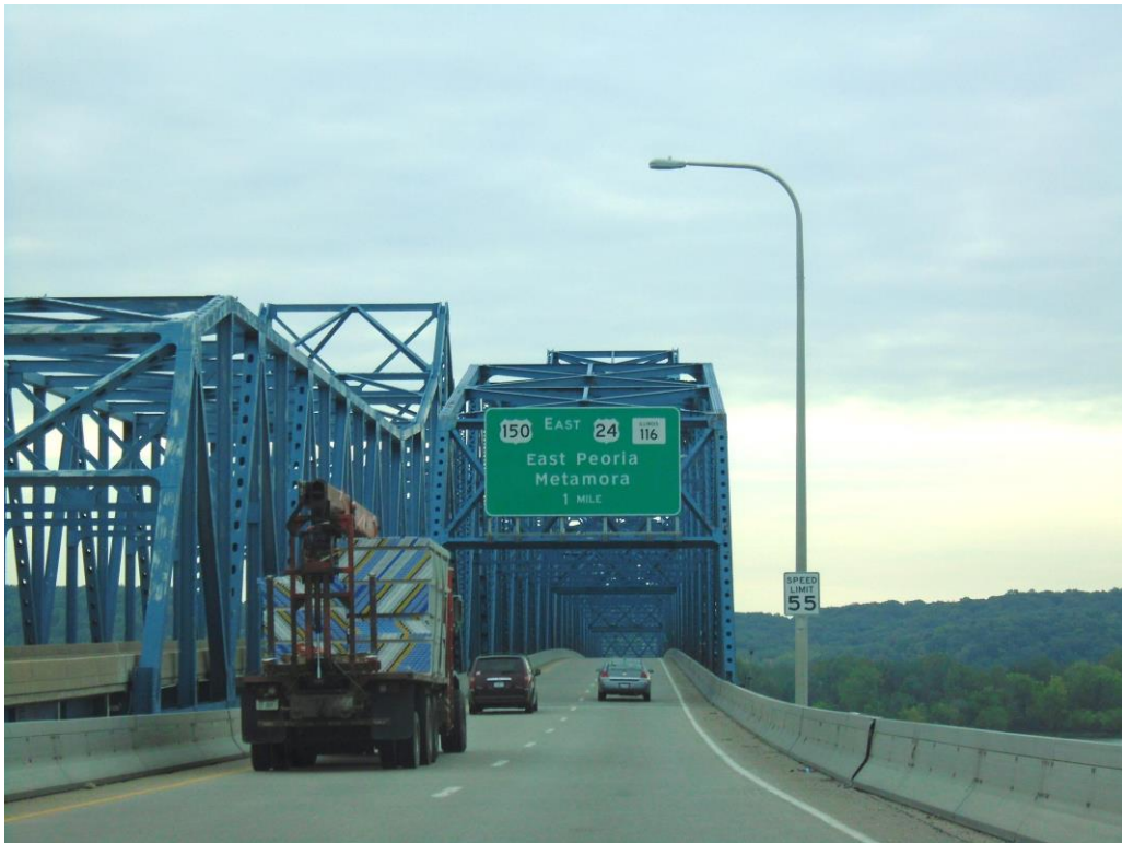
Approaching main bridge span of eastbound US 150 facing east
