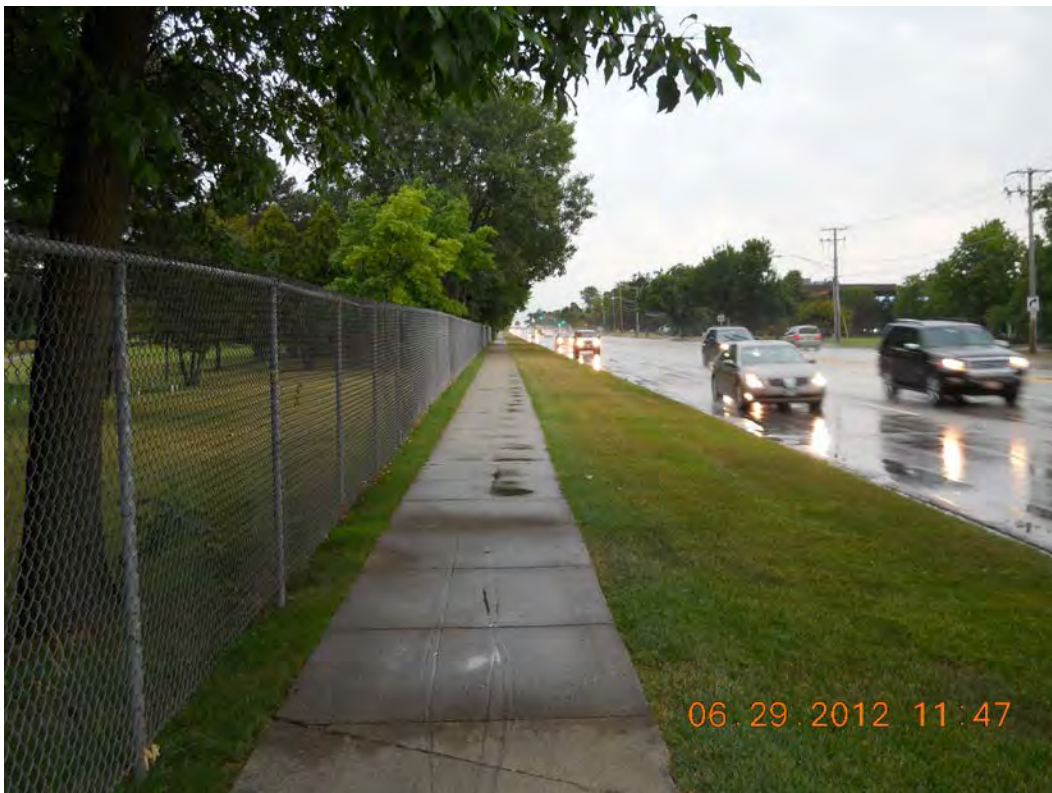
Southwest corner of intersection, west on IL 68 looking west at proposed right turn lane location.
