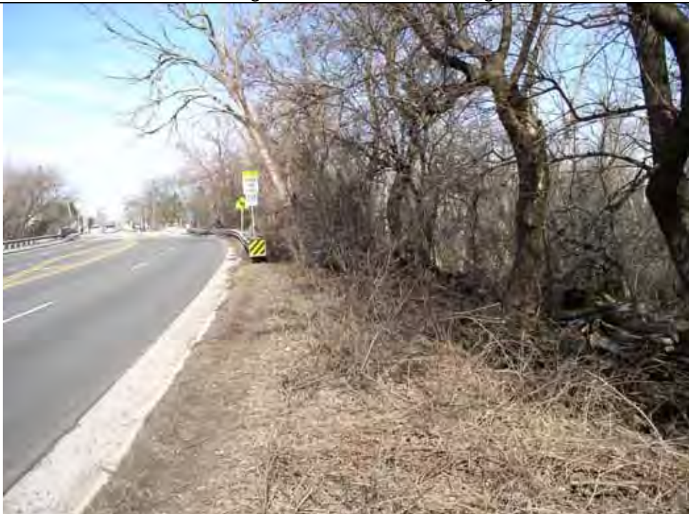
Photo 02 – FPDCC Big Bend Lake Woods located north of Rand Road. Looking West to Rand Road Bridge approach.
